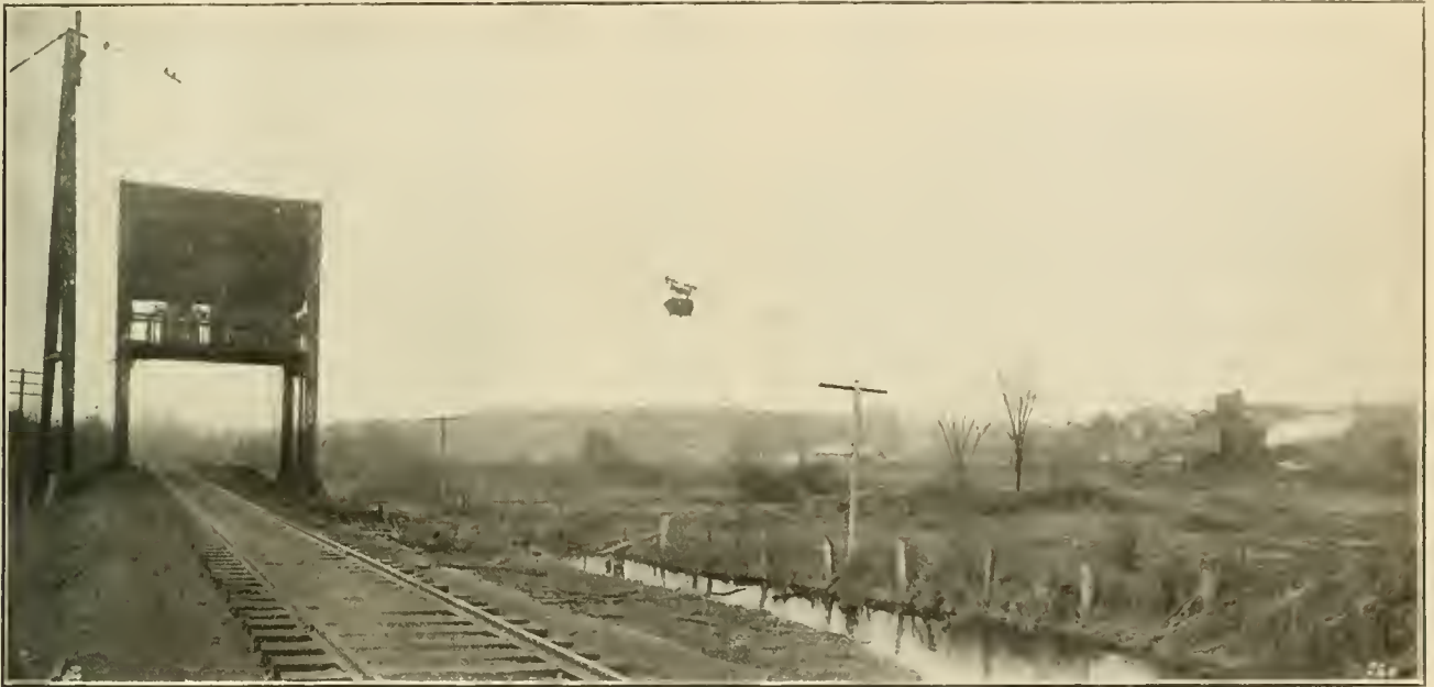
COALING STATION SUPPLIED DIRECT FROM MINE BY TELEPHERAGE CAR.
